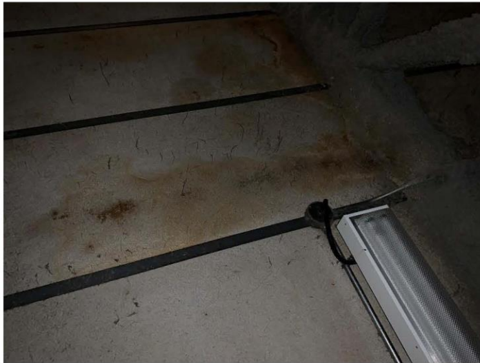
Photo No. 1: Localized Water Damaged Tectum – Above Auditorium Upper Catwalk
