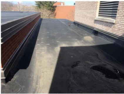
Photo 2 Dirt indicates potential ponding areas
