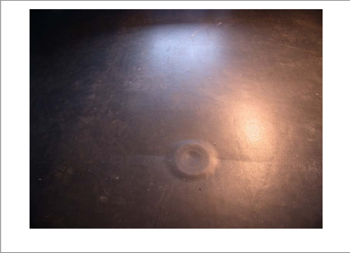
Fig. D.4.2.2-1. Crease in single-ply roof cover while subjected to uplift pressure
