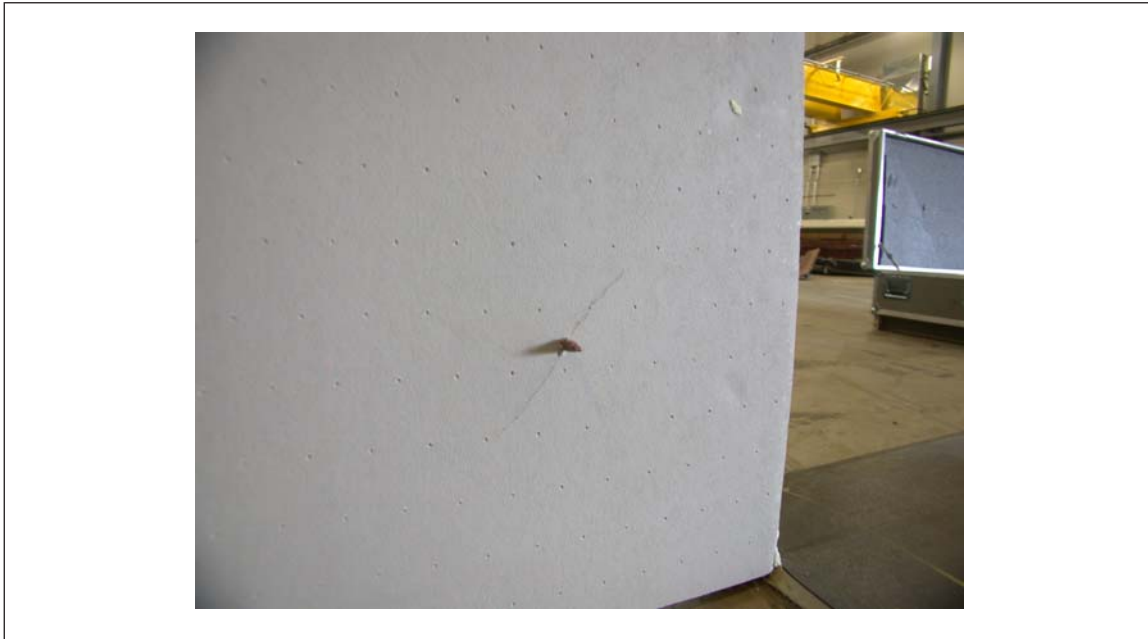
Fig. D.4.2.2-3. Crack in underside of cover board at fastener and beneath where crease was visible in the single-ply roof cover
